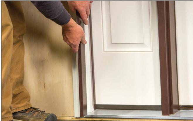
**c. For Single Sidelite Units:** Gently remove the jamb cover out of the utility strip starting at the bottom of the unit and work your way to the top. Repeat for the other side. Next, open the door and remove the door jamb cover by pulling the bottom out from behind the weather strip towards the center of the door working towards the top of the unit.
