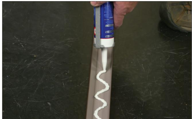
**B. Place the cover over the brickmould, making sure the brickmould cover fits over the jamb cover tabs, and apply pressure from top to bottom ensuring the adhesive bond to the brickmould.**
