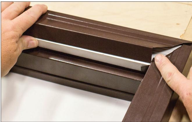
**C.** Apply pressure across the length of the head brickmould cover to ensure the adhesive bond to the brickmould.
