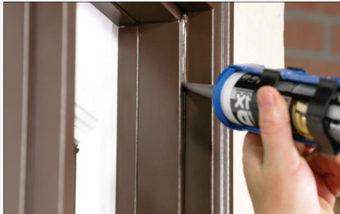
**B.** Repeat step **A** for the other jamb cover, head brickmould cover, and where the mullpost casing covers meet the mullpost jamb covers.
