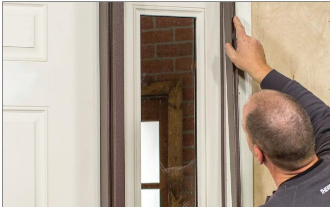
**B. For Single Sidelite Units:** Starting at the top of the unit, gently slide the sidelite jamb cover into the utility strip working towards the bottom of the unit until completely inserted. Next, apply a  $\frac{1}{4}$ " bead of contractor-grade adhesive in a "wide-S" pattern along the inside length of the door jamb cover.
