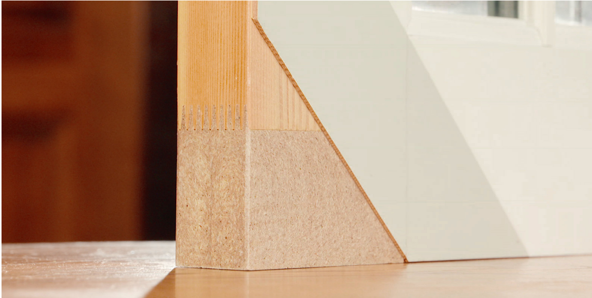
Medium Density Overlay over exterior side of door
