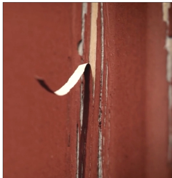
Door with veneer delamination
